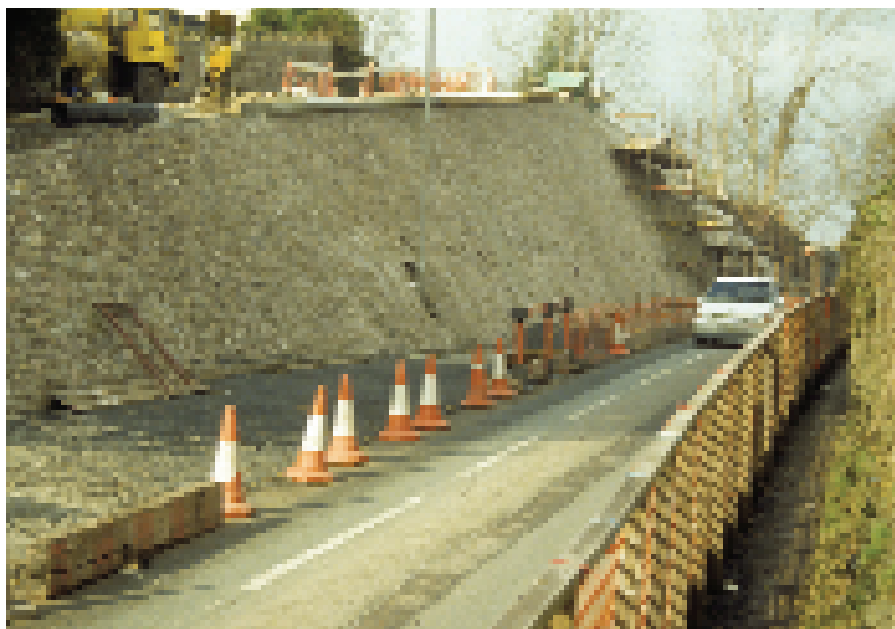
The Cutting at Bwlch was widened in the late 1990s - Chris Barber
